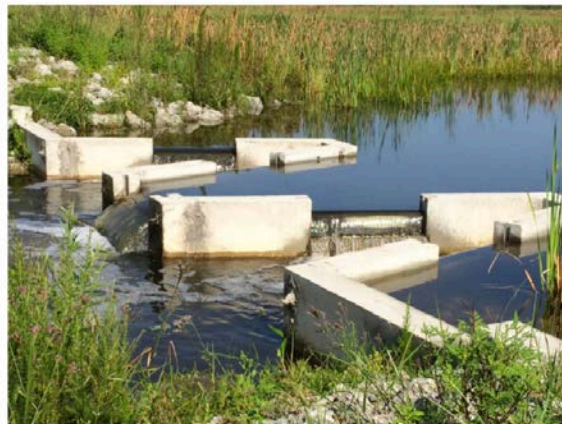
Fig. 3. The labyrinth weir used as the flow control structure at the Cell B Outlet.
